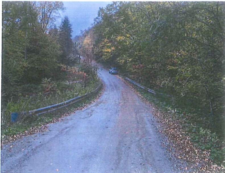
Photo 1 (25) General Topside View (looking east)
